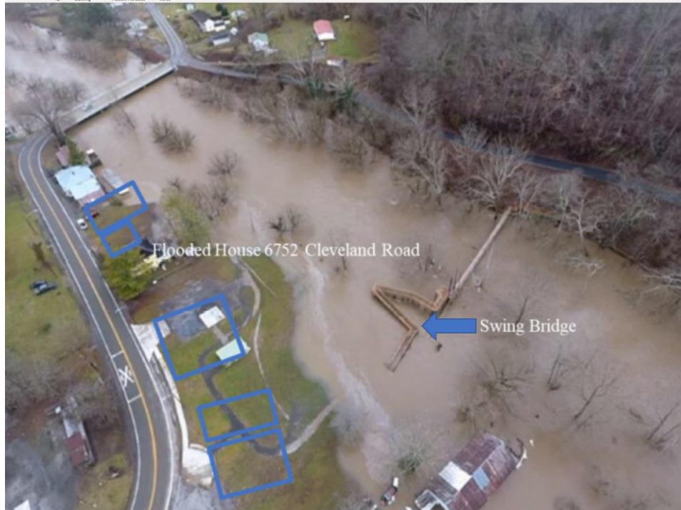
Figure 5: Image of mitigated property parcels flooded in February 2020 rain/flood event
