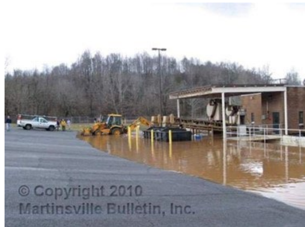
Figure 7: 2010 flood event (peak flood depth approximately 18 inches above grade)
