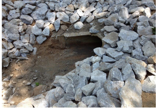
Figure 5: Stormwater fallout maintenance
