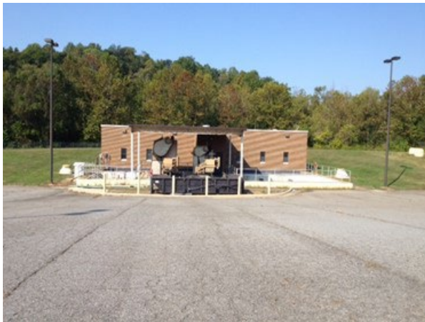
Figure 6: Pretreatment and pumping facility
