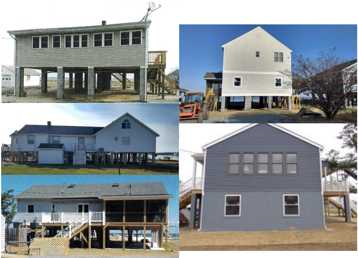
Figure 3: Mitigated properties post-mitigation photos
