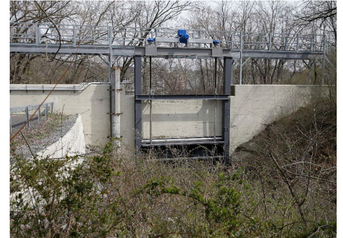
Bowman Dam sluice gate
